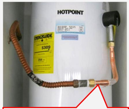
1 flex line is allowed, never 2 connected together, wrong slope
