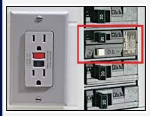
GFCIs are sometimes in electrical panels but most often in outlets. The GFCI works by measuring the difference in currents flowing in the hot and neutral wires.
